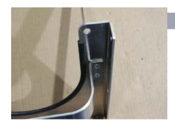
Rivet second Face Plate to Main Bracket.
